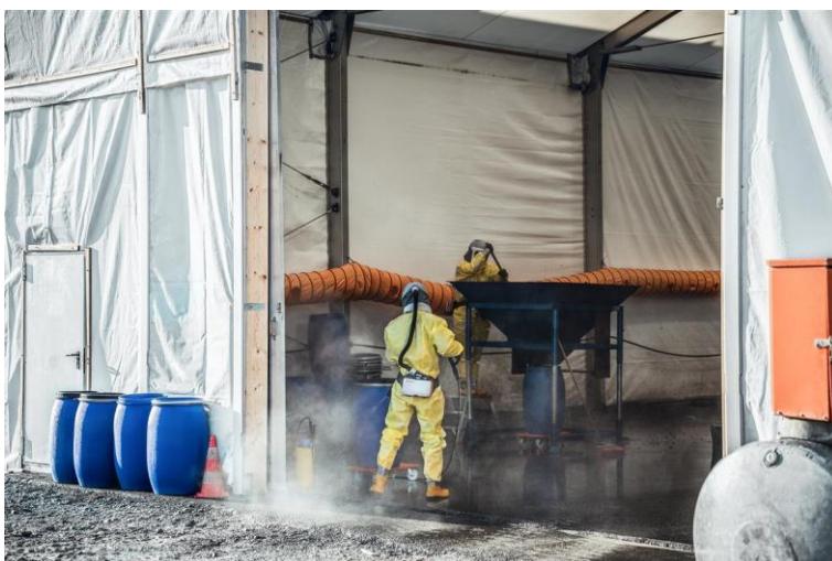
(2) Special protective suits and an exhaust air purification system ensure the safety of employees and environment.
