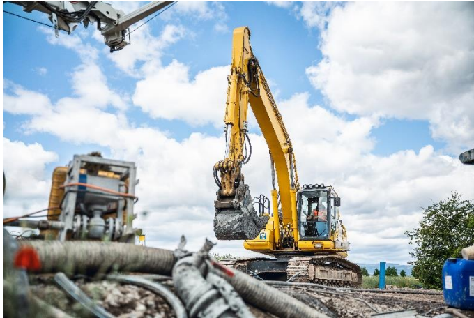
(2) The experienced team laid more than 10,000 m of pipeline.
